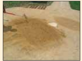
Cover with a thin layer of infield mix to finish grade.
