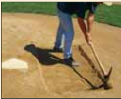
Excavate the Batter's Box 3" deep.
